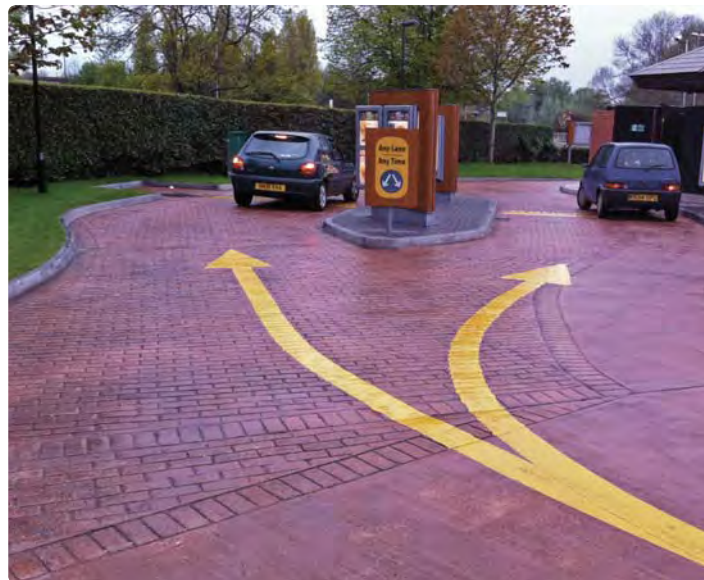
Above: Winner of the Commercial Installations category – McDonald's restaurant drive-thru lanes, Cosham in Portsmouth.
