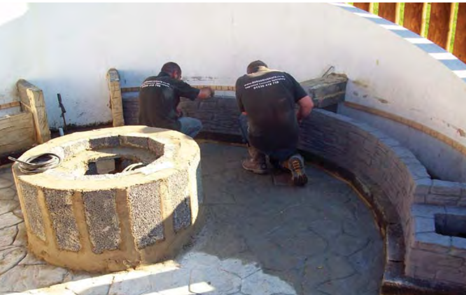
Above: Construction of a fire pit.
